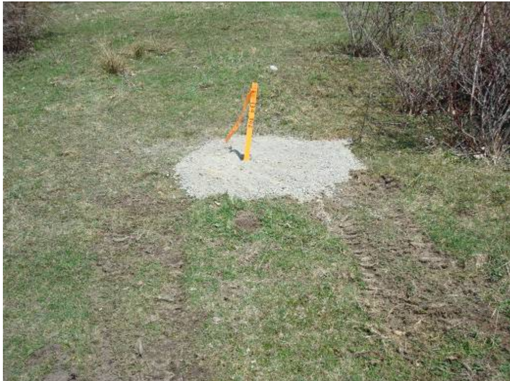
Picture C-6: Drill cuttings surrounding drilled shot hole.
